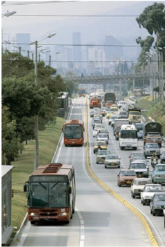
Fig. 1 Bogotá TransMilenio BRT system.
